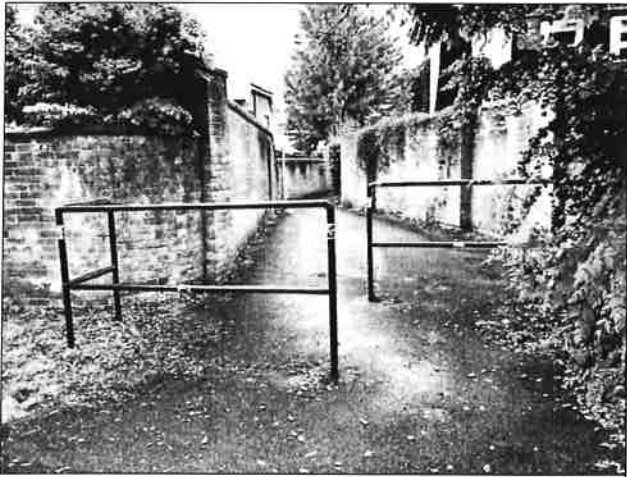
The barrier at The Harrage onto Southampton Road. Wide enough for everyone.
